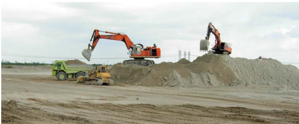
Figure 40: Mining operations at the Palm Beach Aggregates mine within the Palm Beach County Limestone Resource Area (Source: LHC)
