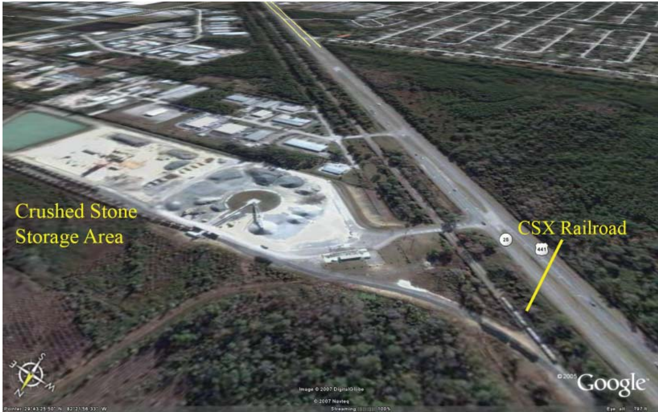
Figure 17: Conrad Yelvington Distributors, Inc. terminal at Gainesville, Florida, which illustrates a typical design and layout
