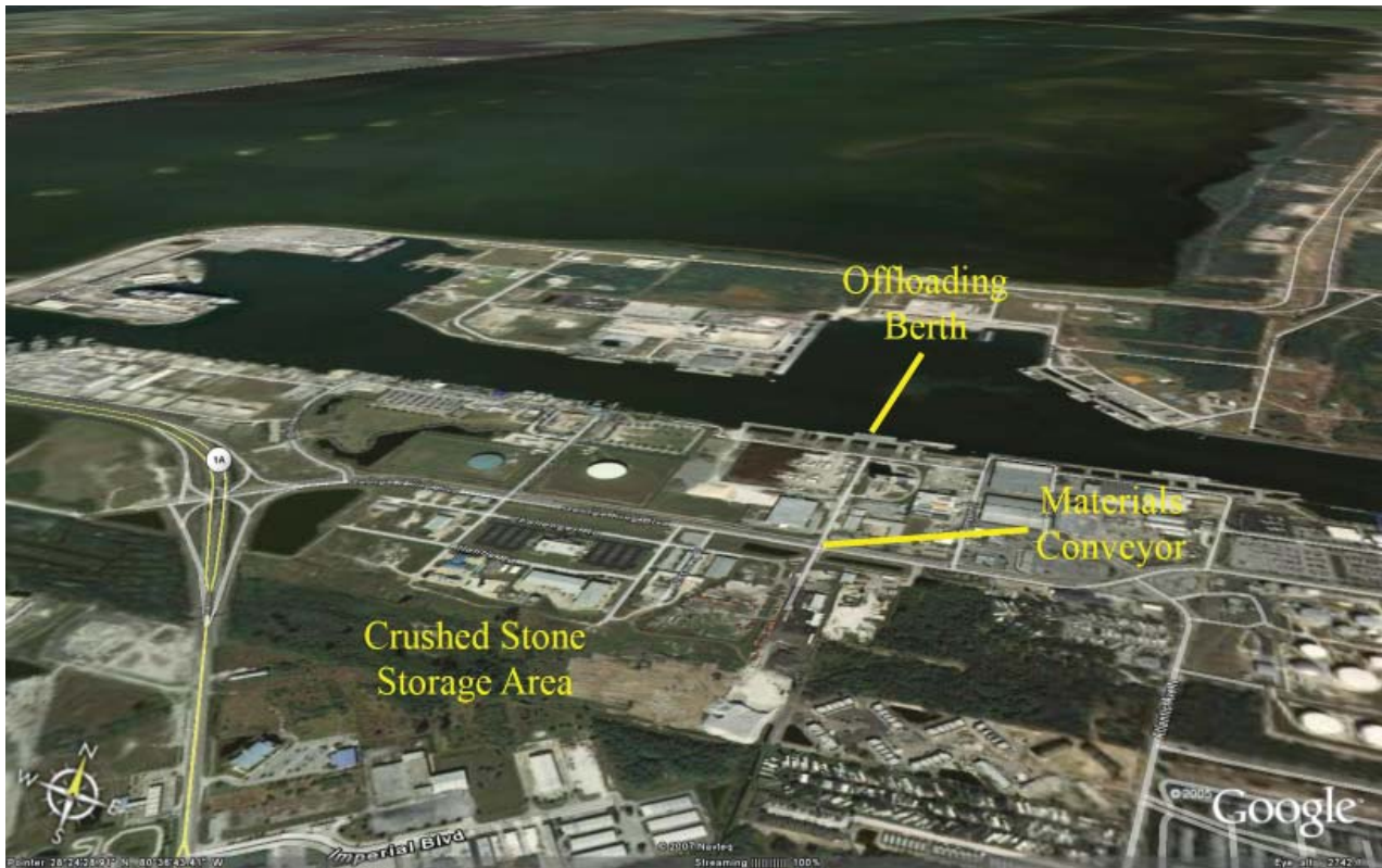
Figure 22: Berthing and terminal facilities at Port Canaveral.
